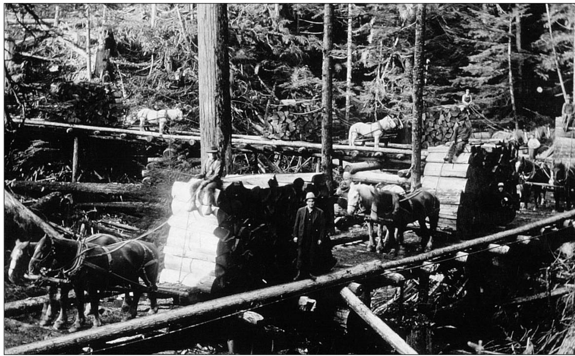
Horse-drawn sledges haul shingle bolts along a trestle bridge on a logging skid road in the Seymour Range in 1915.
